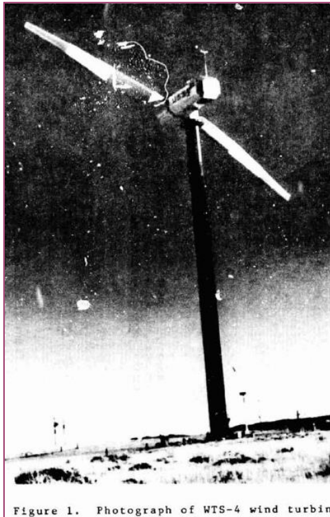
Figure 1. Photograph of WTS-4 wind turbin
